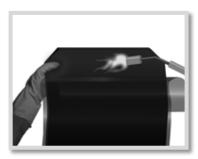
Step 7: Partially remove the release liner from the sleeve ( $\sim$ 6" from the edge) and gently heat the adhesive along the underlap with a torch.
