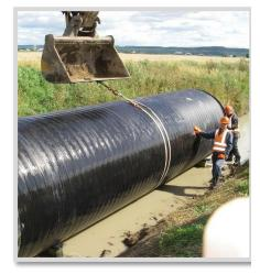
Step 3: Use nylon slings with lever or excavator arm to rotate the pipe.
