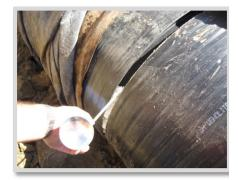
Step 1: Thread pipe together until 1 complete turn is remaining to complete threading.
