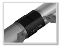
Step 18: As a final check, ensure that the sleeve follows the entire contour of the surface and that there are no cold spots or burning of the sleeve. Make sure the edges of the sleeve are not lifting anywhere around the circumference of the pipe. This can be checked by feeling the edges all around the circumference of the sleeve. If there is edge lifting, the edge should be reworked with additional heat.
